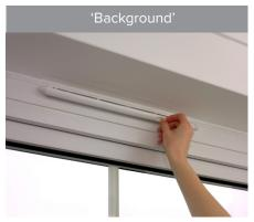
A small ventilation opening designed to provide controllable whole dwelling ventilation.
